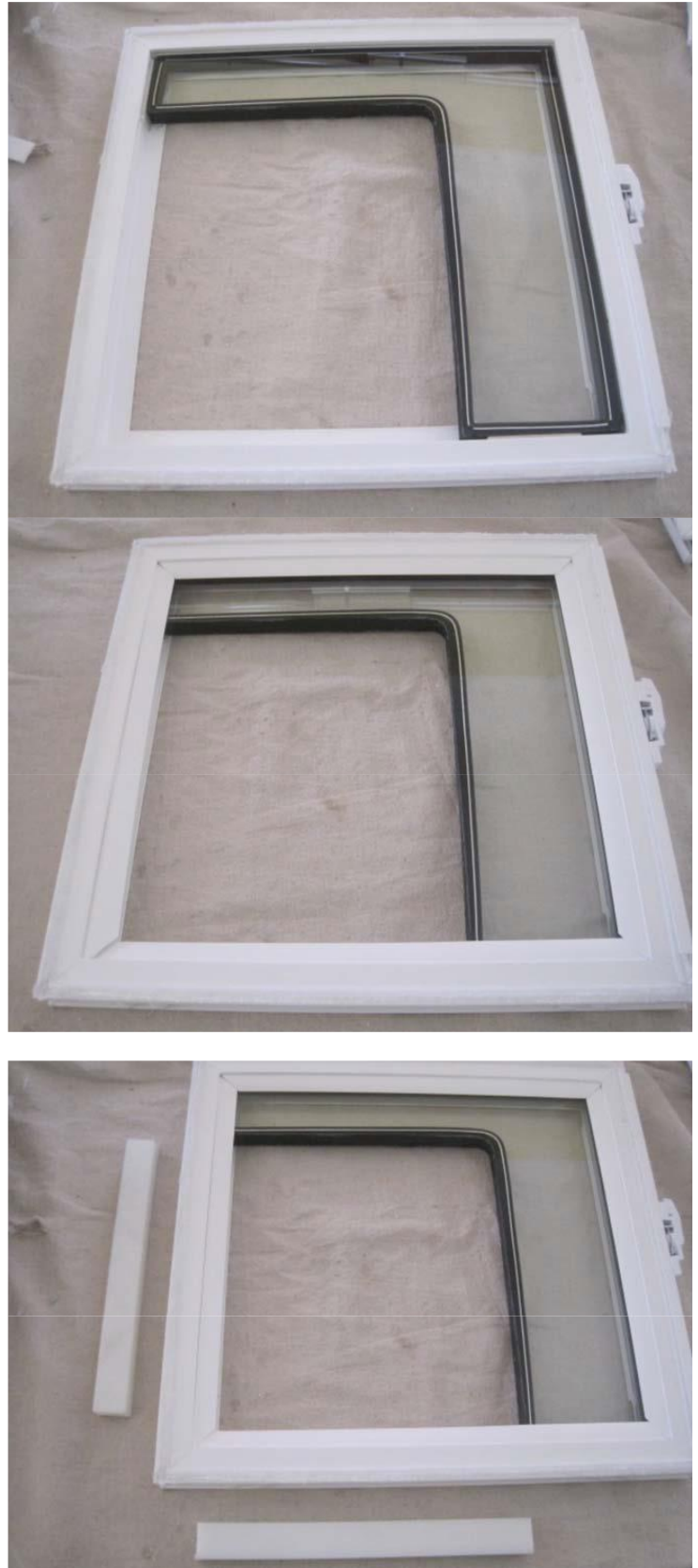
Figure 4 New IG Unit installed in door panel
