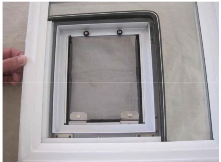
Figure 8 Gap clearance between pet door and glass
