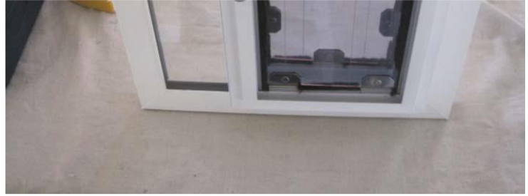
Figure 9 Pet door installed in door panel
