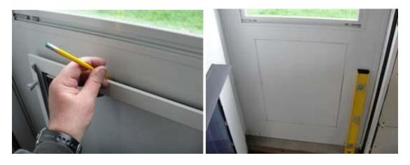
**Step 5—WOOD DOORS:** For wood doors, drill out two corners diagonal from each other using a 7/8" paddle bit or a 5/16" regular bit. If you use a regular bit, drill three holes close together then elongate the holes until you have connected the three holes. This will allow insertion of the reciprocating saw blade. Cut out the rough opening along the traced lines.
